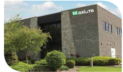
(HQ) West Caldwell, NJ
